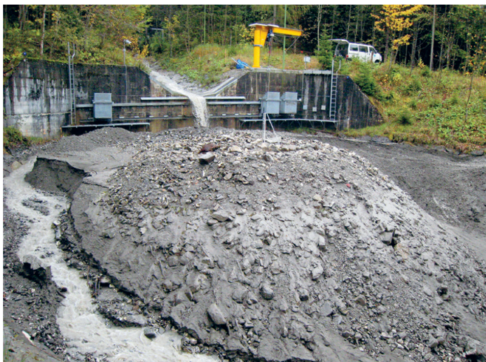
The sediment transported by the Erlenbach during flooding collects in the inlet basin. It is measured regularly and then dredged.
